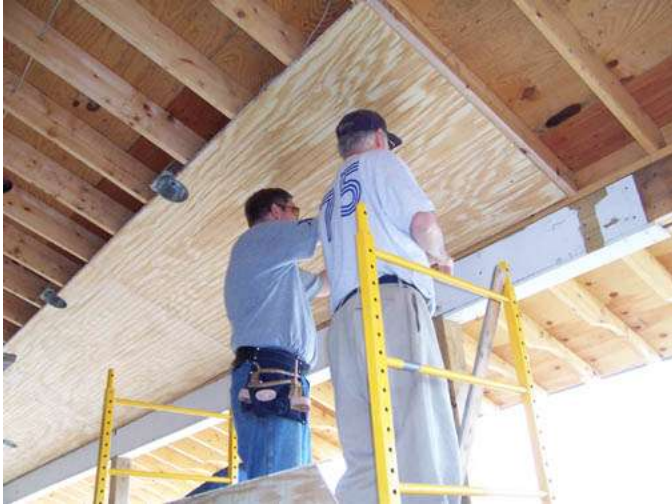
Installing Beadboard Under Porch Roof (JB)
