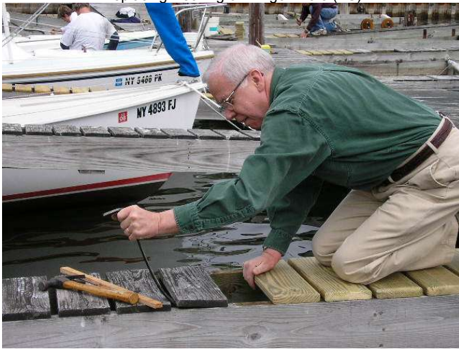
Replacing Decking on Finger Piers (AS)
